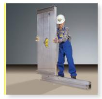
Should you require a trench box, just guide the number of plates you need into the corner posts.
